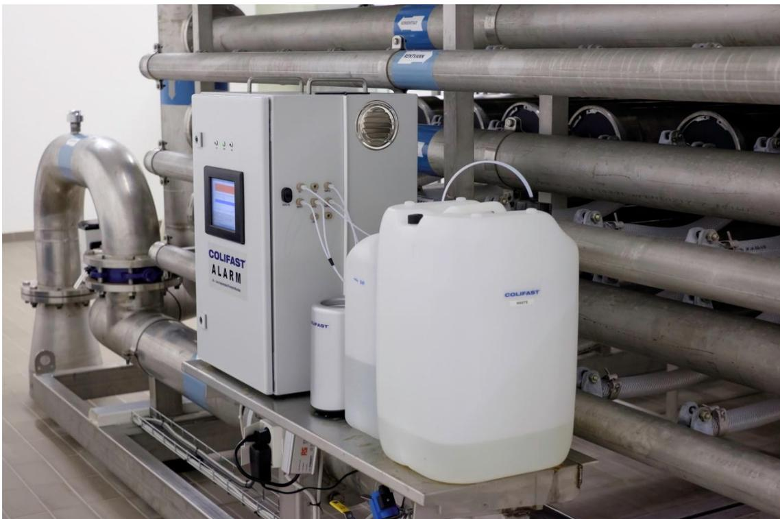
The Colifast ALARM monitoring the drinking water produced at a drinking water treatment plant
